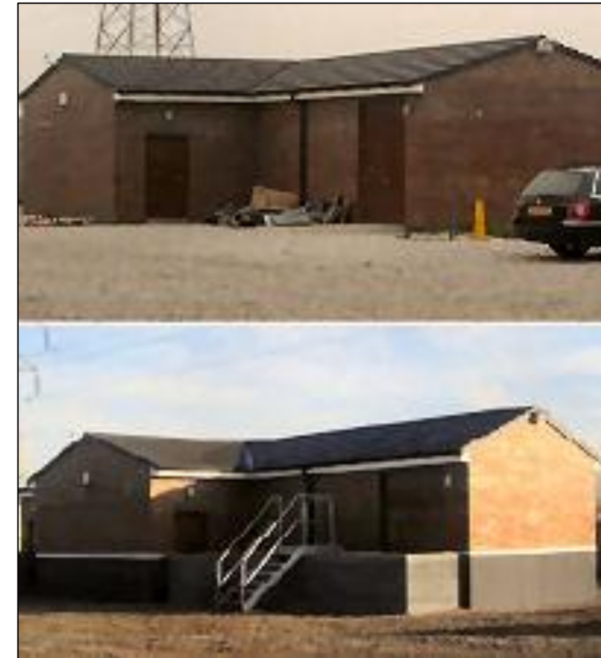
Figure 6.11: Veneer walling and access steps
