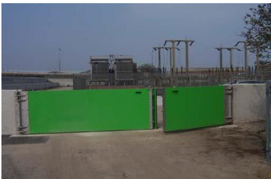
Figure 6.6: Flood protection gates (ENA ETR138 Annex 1)
