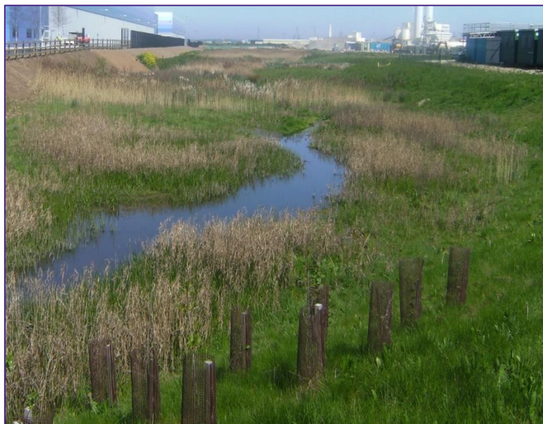
Figure 2-1 Detention Basin with low flow channel
