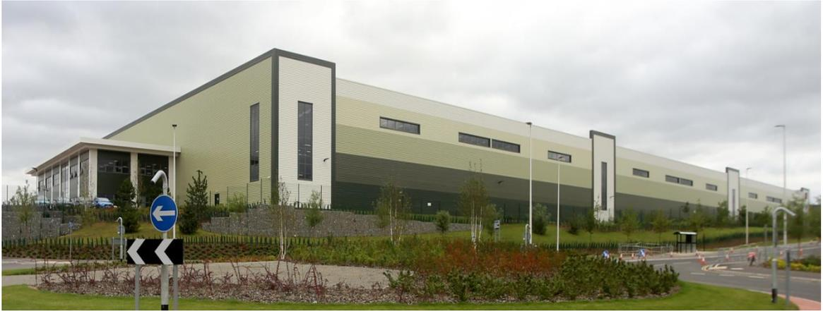
**Figure 12: Use of colour banding to reduce visual mass**
