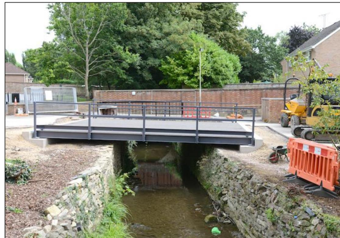
Figure 3.1: Example of temporary span bridge
