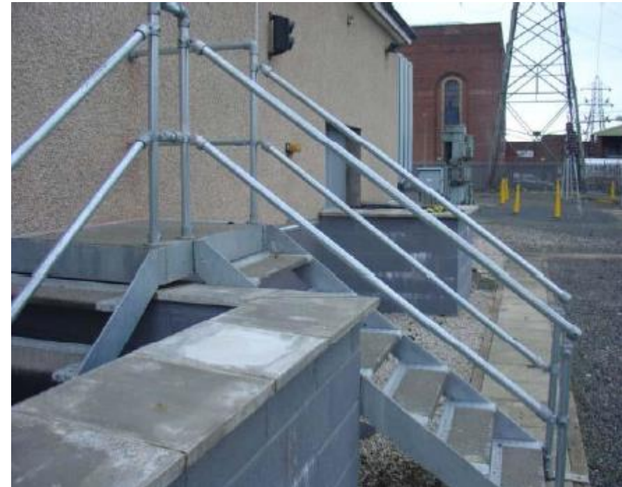
Figure 6.3: Access to Substation entrance (ENA ETR138 Annex 1)
