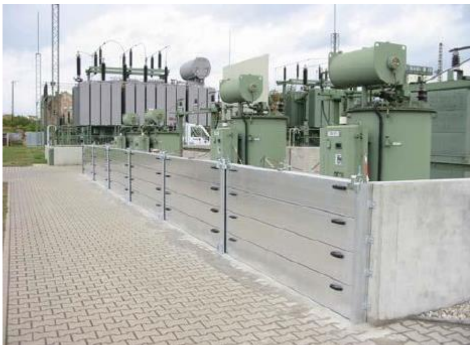
Figure 6.5: removable flood panels (ENA ETR138 Annex 1)
