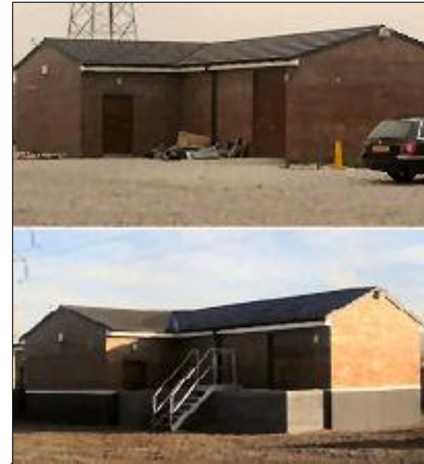
Figure 6.11: Veneer walling and access steps
