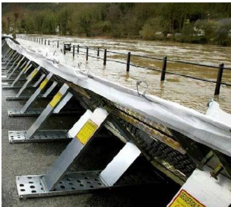
Figure 6.10: Temporary flood defence system (ENA ETR138 Annex 1)
