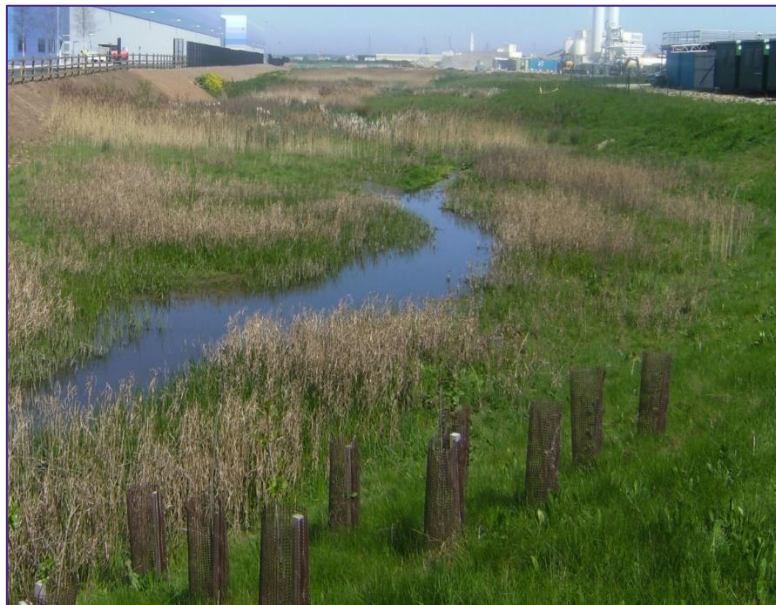
Figure 2-1 Detention Basin with low flow channel
