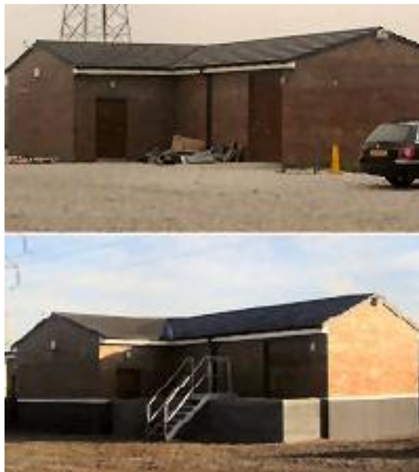
Figure 6.2: Veneer walling and access steps
