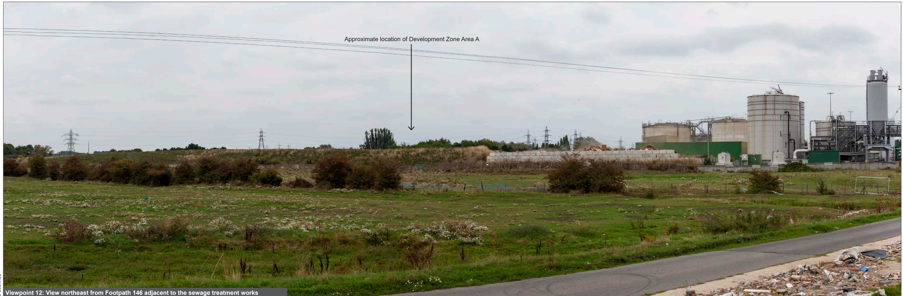
Viewpoint 12: View northeast from Footpath 146 adjacent to the sewage treatment works
